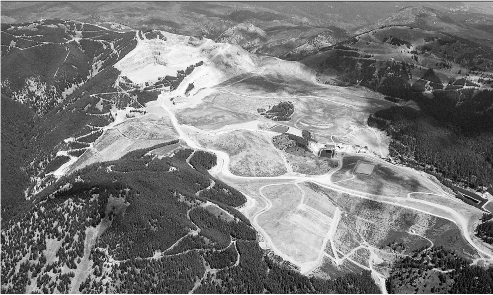
Zortman 2004 Reclamation near completion
